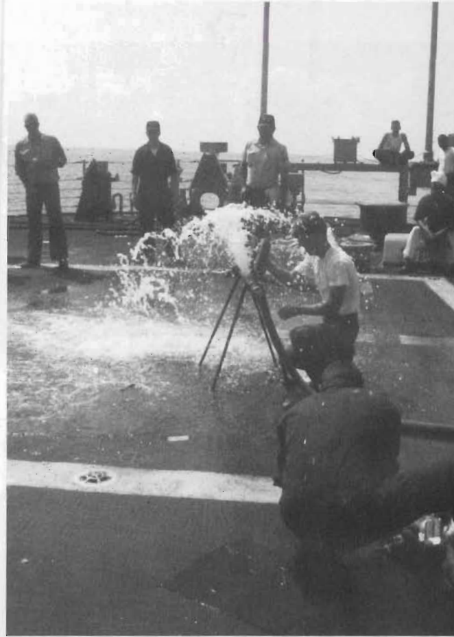
Pipe patching can be a wet job
