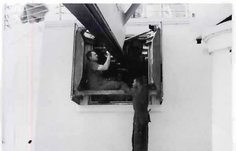
GMM's work on the rails
